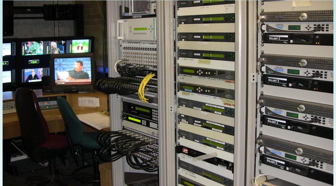
The SABC's DTT playout facility and coding and multiplexing infrastructure
