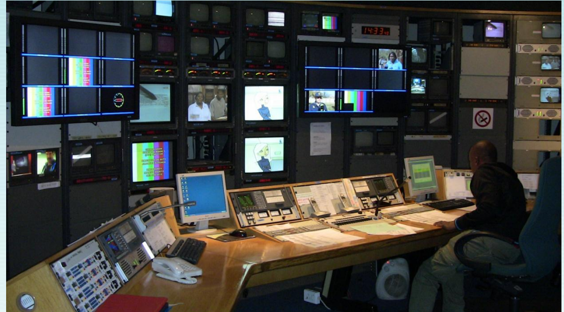
The exiting Master Control Room which is to be replaced with the implementation of the new Digital Playout Centre
